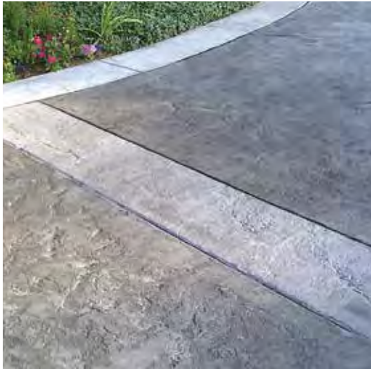
Heavy Stone Texture Skin Stone Gray Color Hardener (border) / Light Gray Antique Release
