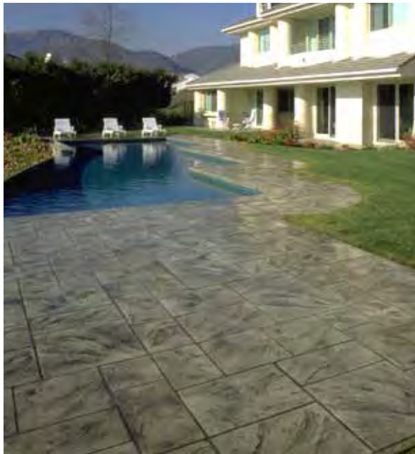
36" Ashlar Cut Slate Sun Buff Color Hardener / Medium Gray Antique Release
